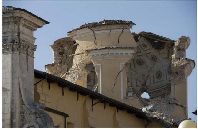
Figure 5. The Chiesa delle Anime Sante dome after the earthquake.
